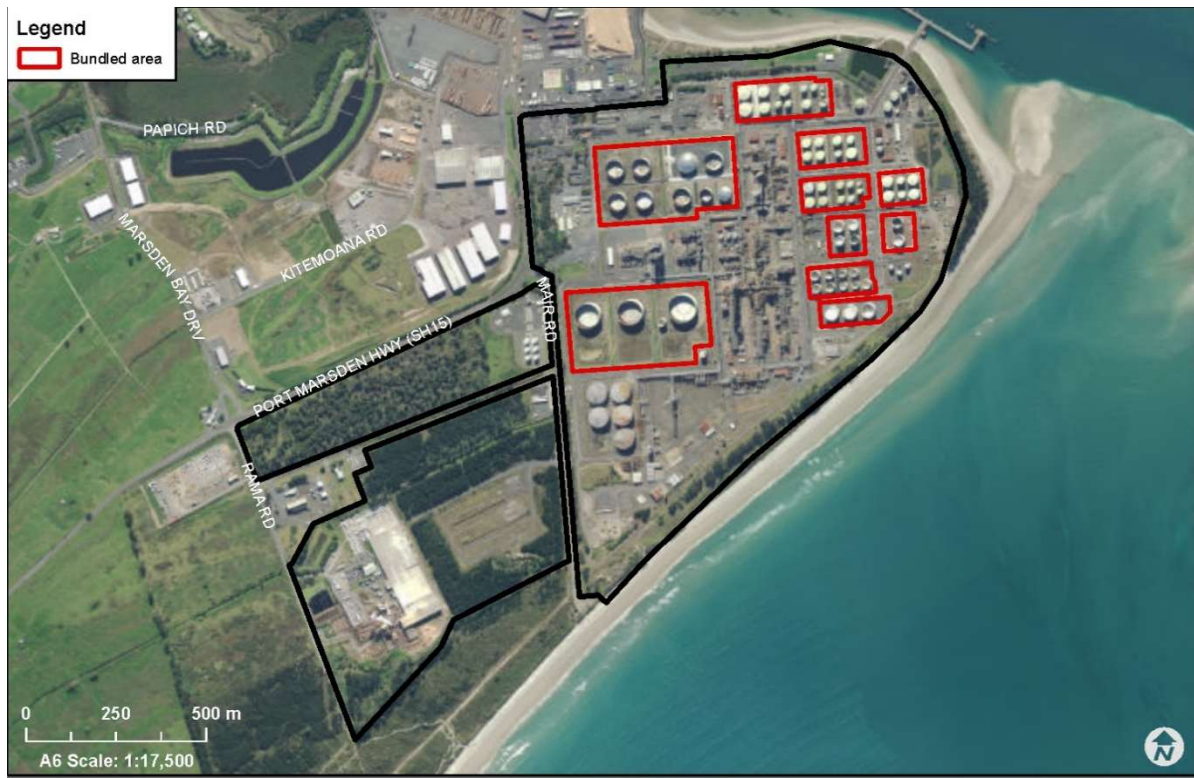
Figure PREC6 1 Bundled Area
