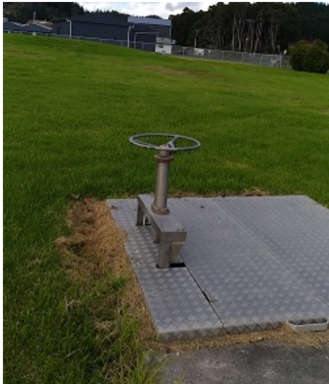
Figure 15 - Emergency outfall isolation valve (with manual padlock)
