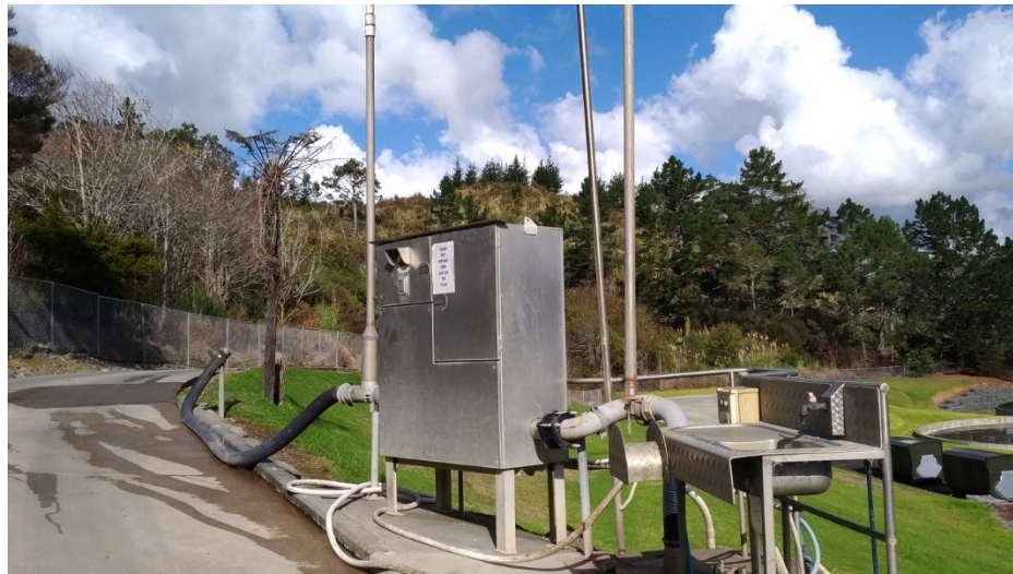
Figure 4 - Septage Receiving Facility
