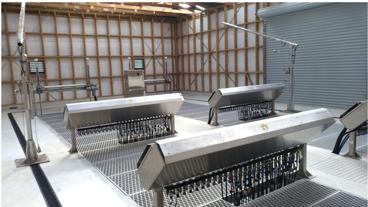
Figure 13 – High Flow UV treatment facility
