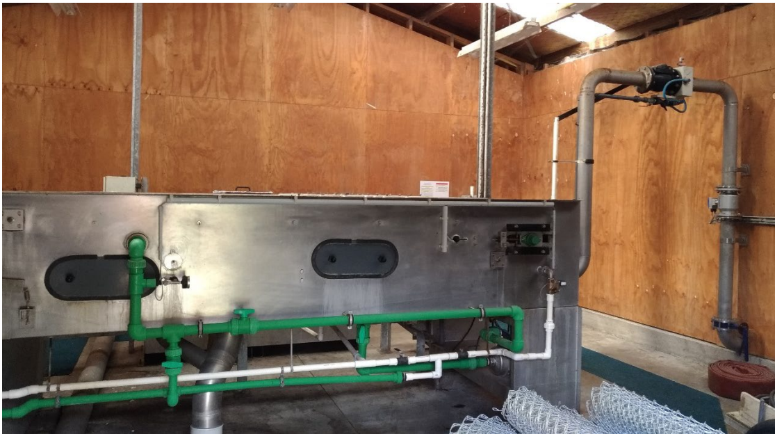
Figure 17 - WAS gravity belt thickener
