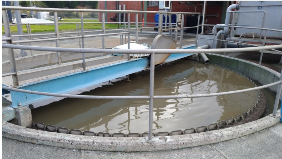
Figure 16 - Primary sludge gravity thickener
