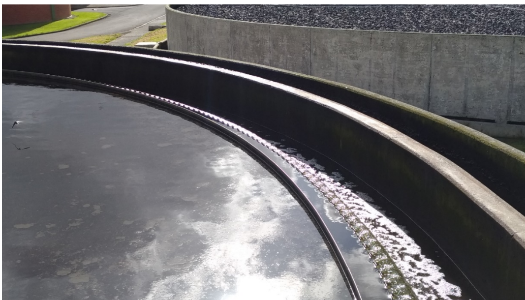
Figure 11 - Secondary clarifier launder
