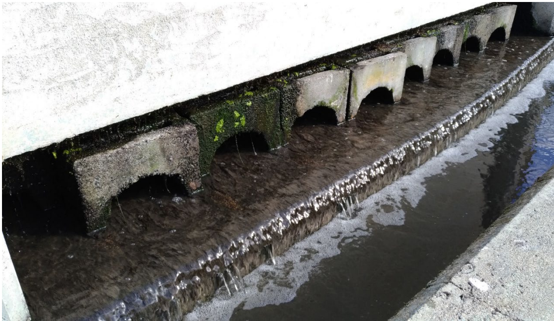
Figure 7 - Trickling Filters – outlet launder
