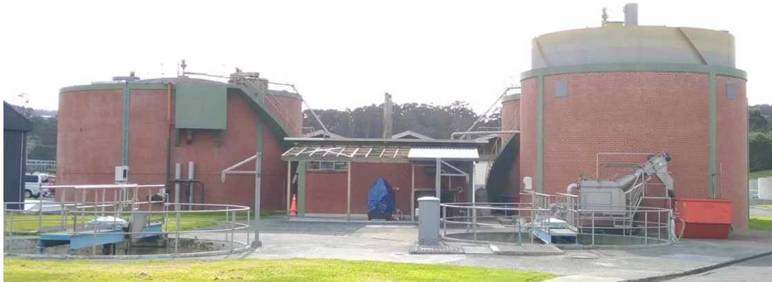
Figure 18 - Digester Tanks and Gravity Thickeners (buried foreground)
