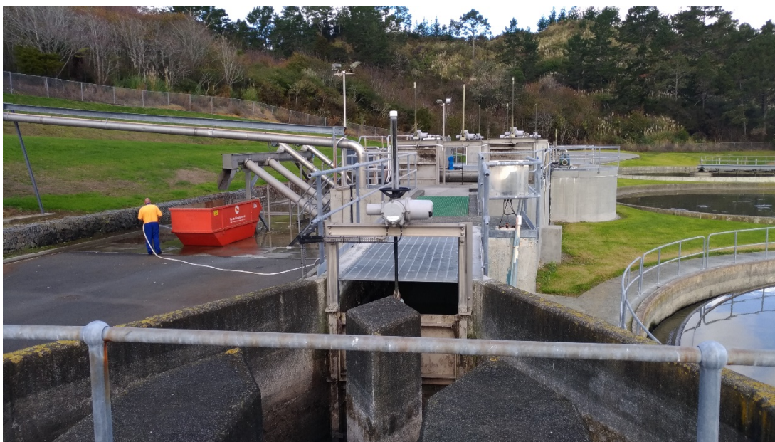
Figure 3 - Inlet Works – view towards the Band Screens
