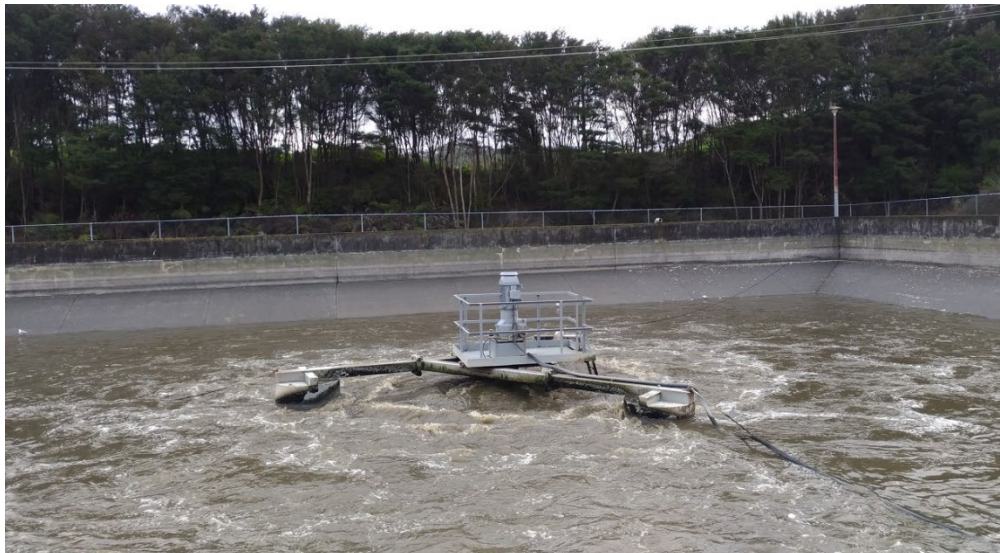
Figure 5 - Equalisation Basin and surface aerator
