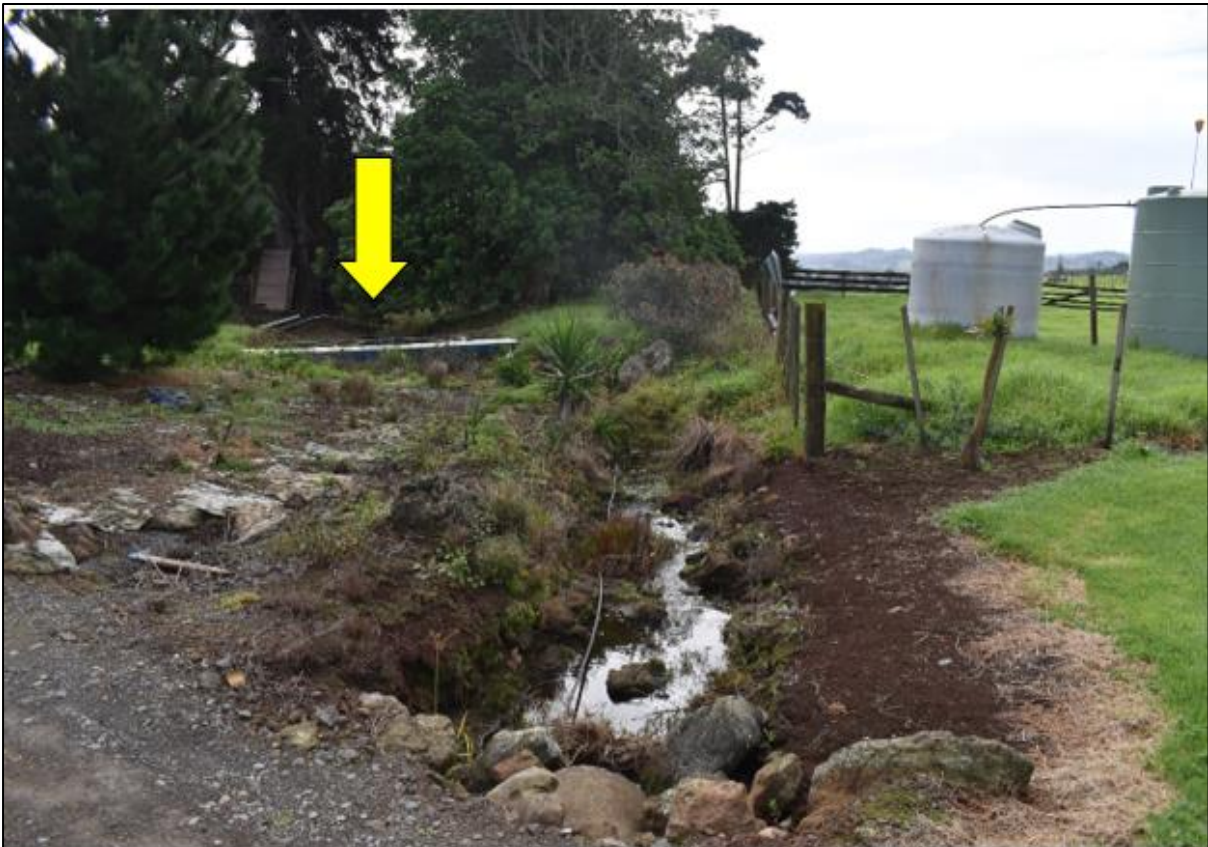
Figure 6: Showing the existing crossing over Waitaua Stream and where the stream seeps into soil and drops for about 10-15m (yellow arrow)
