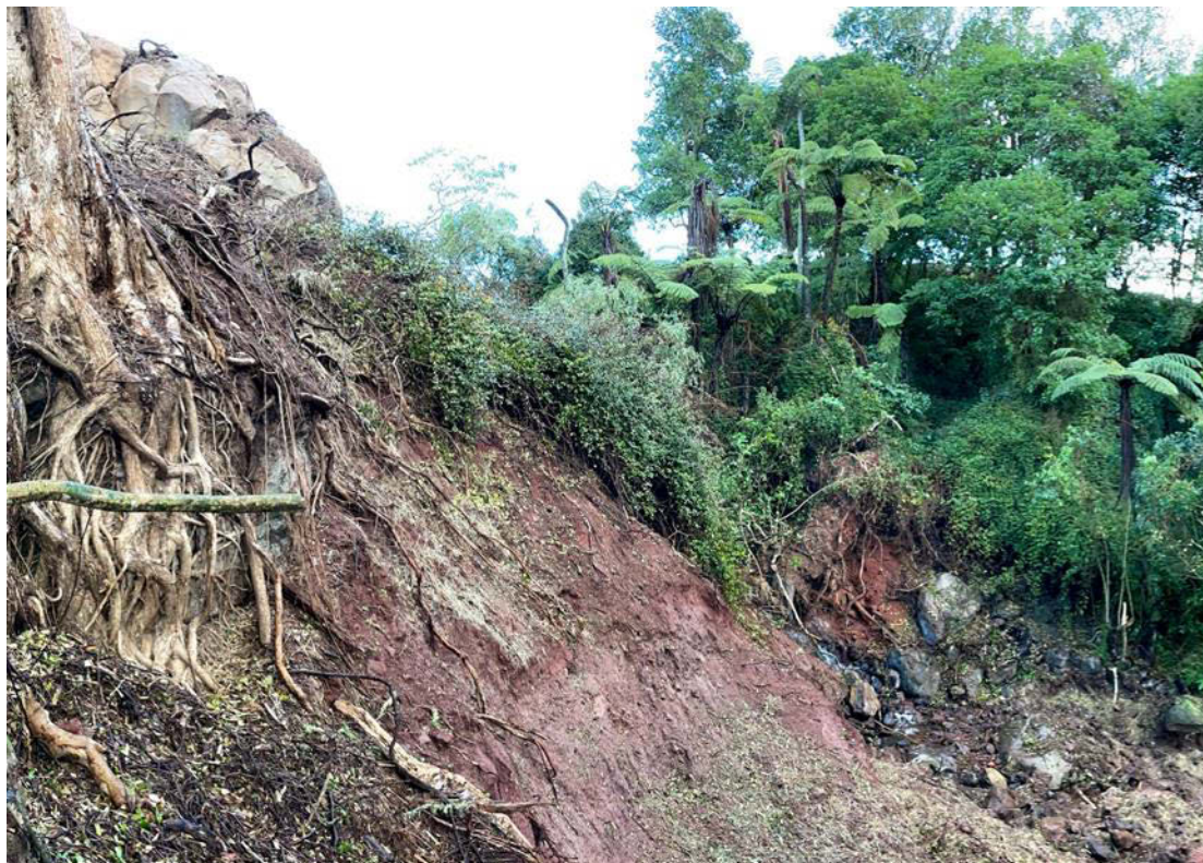
Figure 4: View west across the southern gully slope, showing large basalt promontory at crest of slope (top left), tephra soils immediately below, and boulders of basalt over the gully floor.
