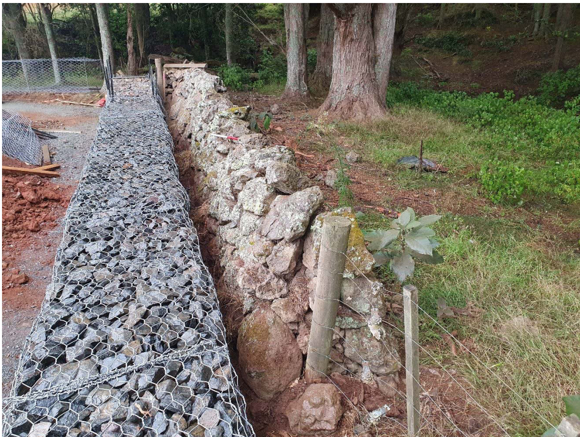
Figure 42: Section of wall in fair condition along northern boundary.
