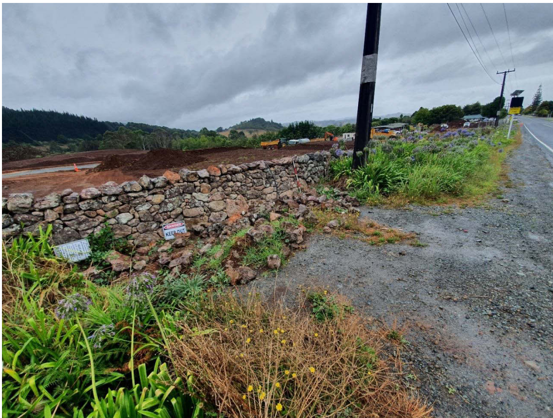
Figure 32: Northern road crossing gate, after infilling.
