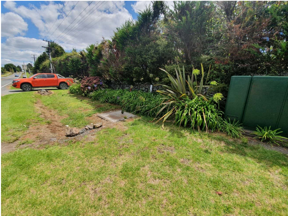
Figure 48: Three Mile Bush Road boundary wall, landscaping and services.
