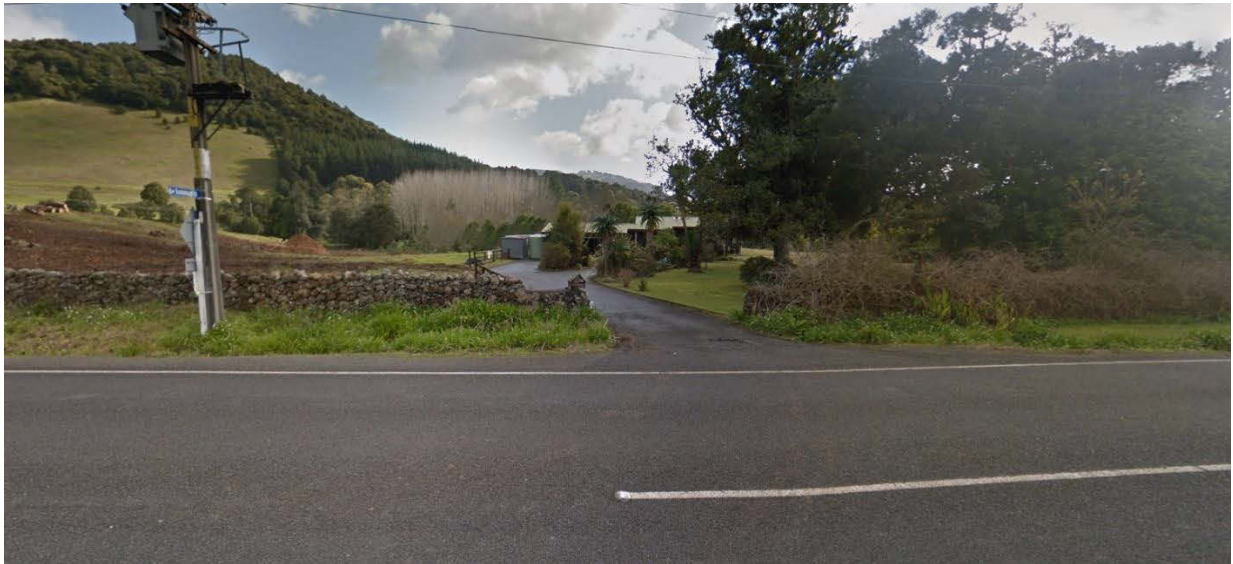
Figure 27: 115 Three Mile Bush Road crossing, prior to works commencing (Google Streetview).
