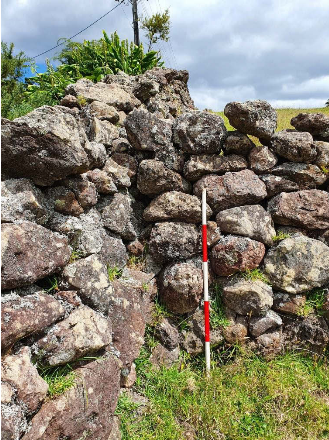
Figure 52; Internal wall built against Three Mile Bush Road boundary wall.
