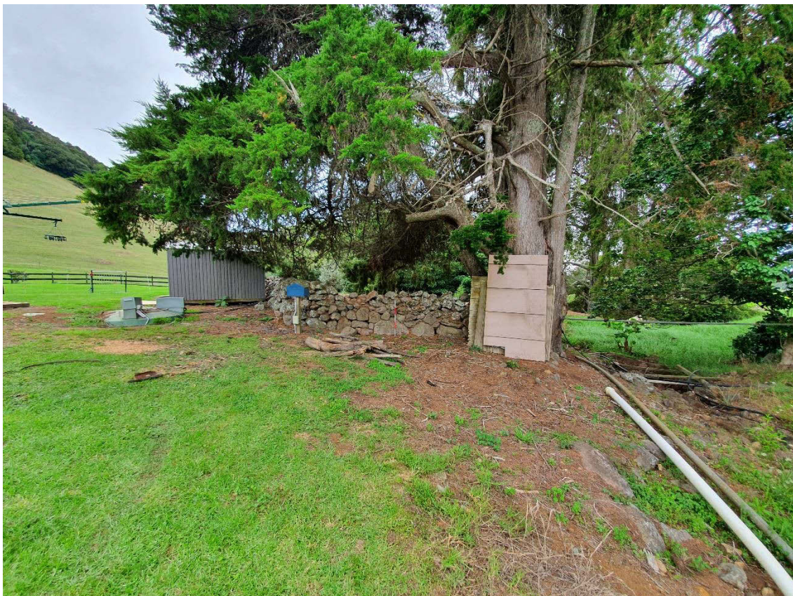
Figure 61: South west end of internal stone wall.
