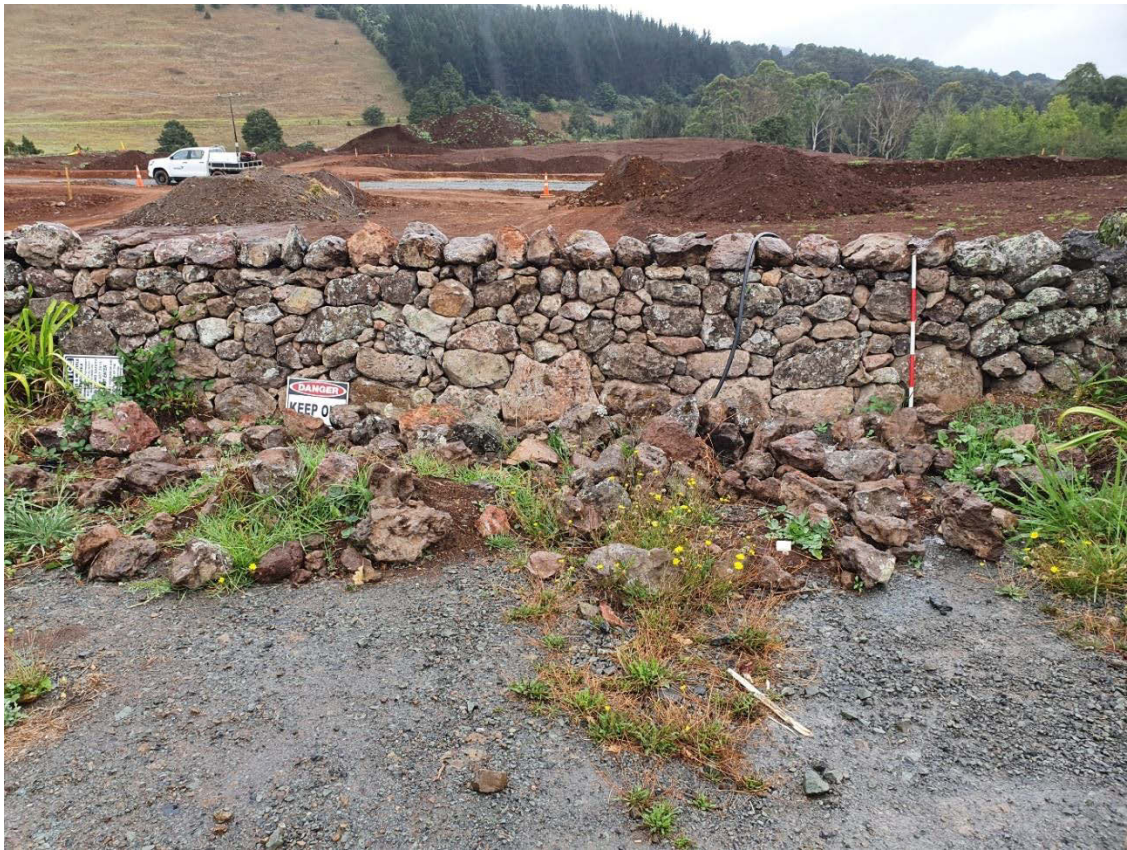
Figure 33: Northern road crossing gate after infilling.
