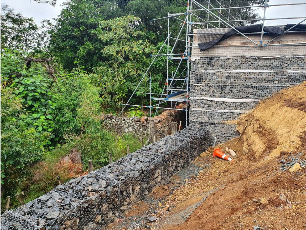
Figure 40: Otapapa boundary wall relocation.
