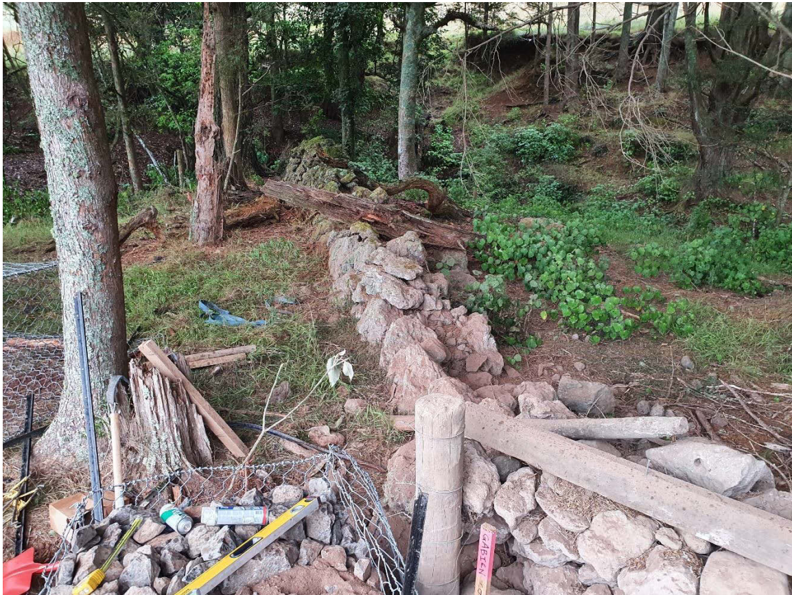
Figure 43: Section of stone wall in poor condition on northern boundary.
