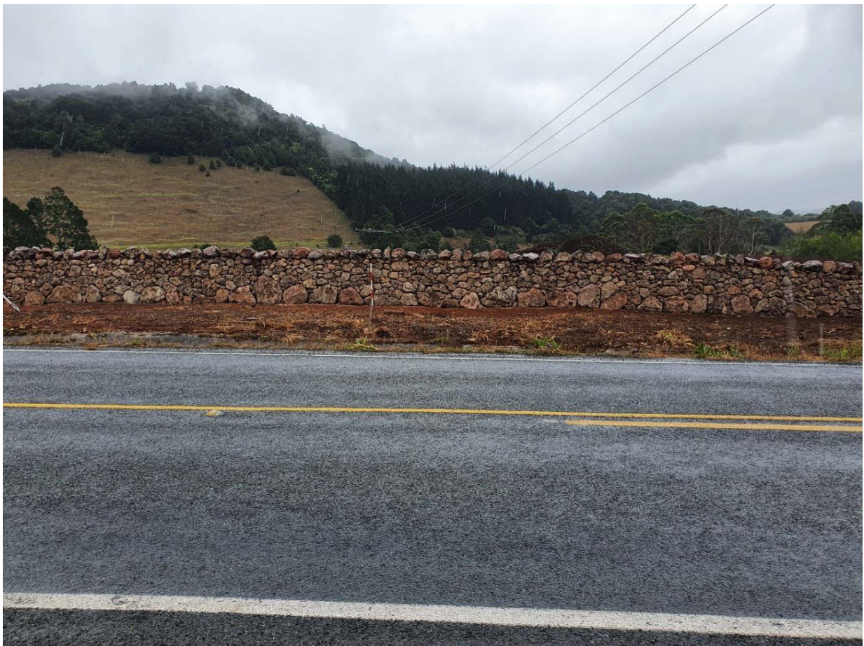
Figure 38: Northern hillock, after re-contouring and relocation of power pole.
