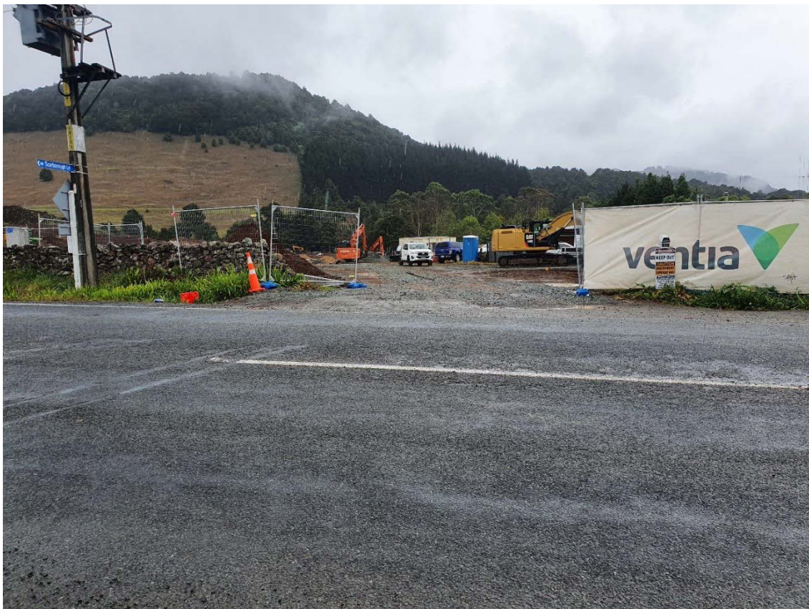
Figure 28: Current 115 Three Mile Bush Road crossing, to be closed.
