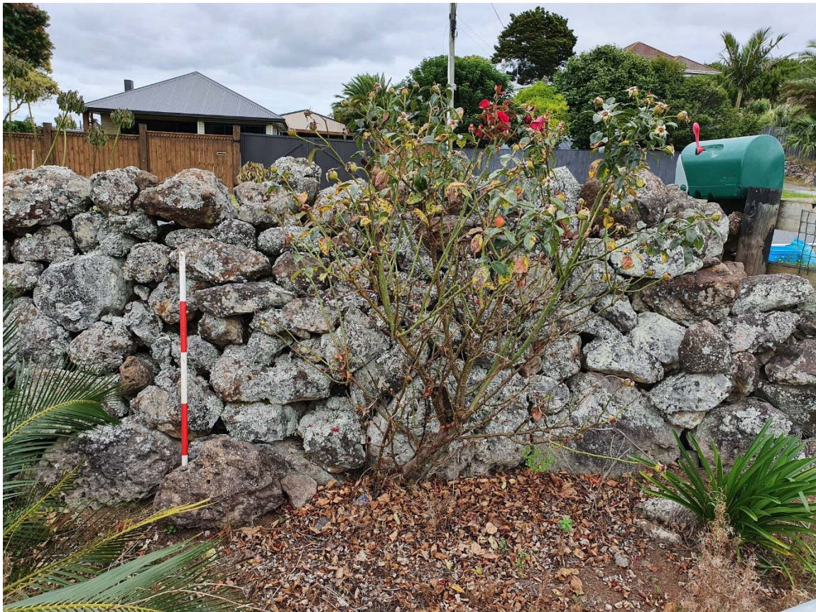
Figure 60: Detail of stone road boundary wall adjacent to road crossing.
