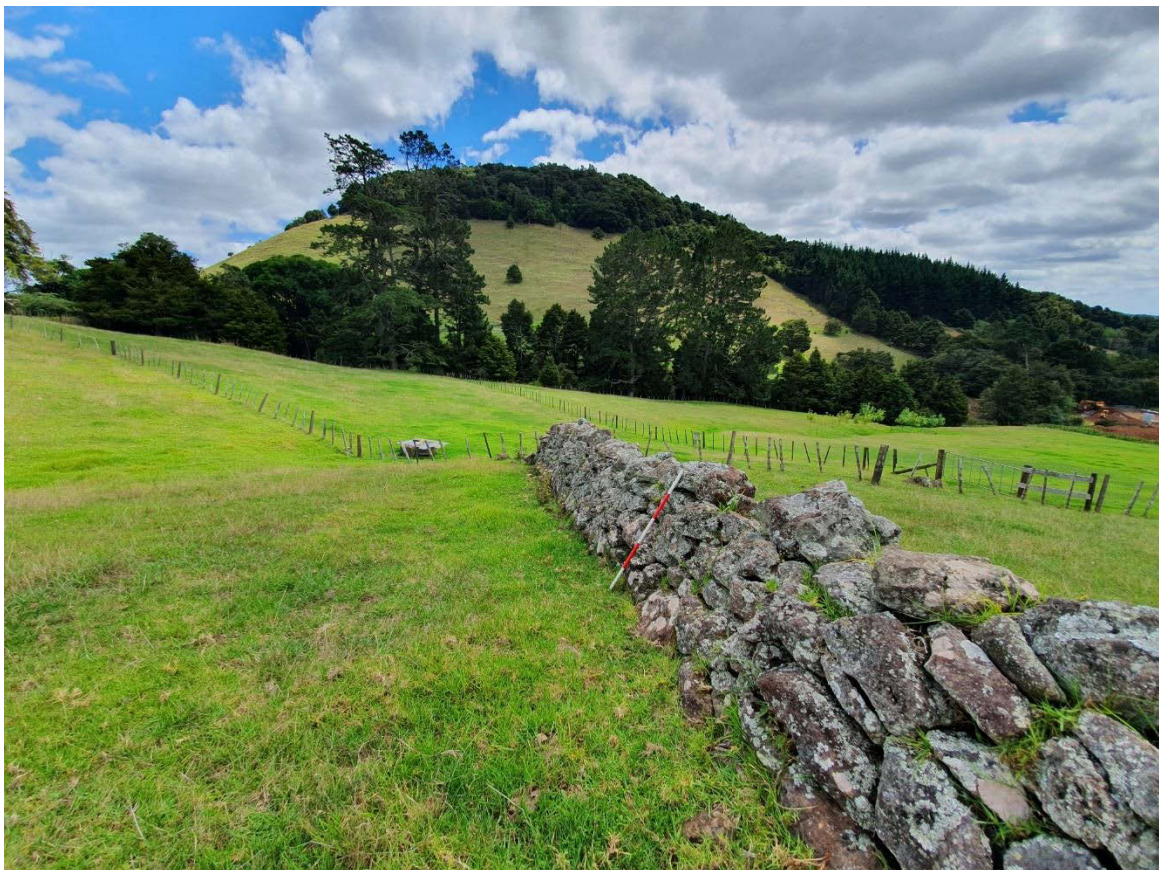
Figure 55: Northern termination of wall, looking north.
