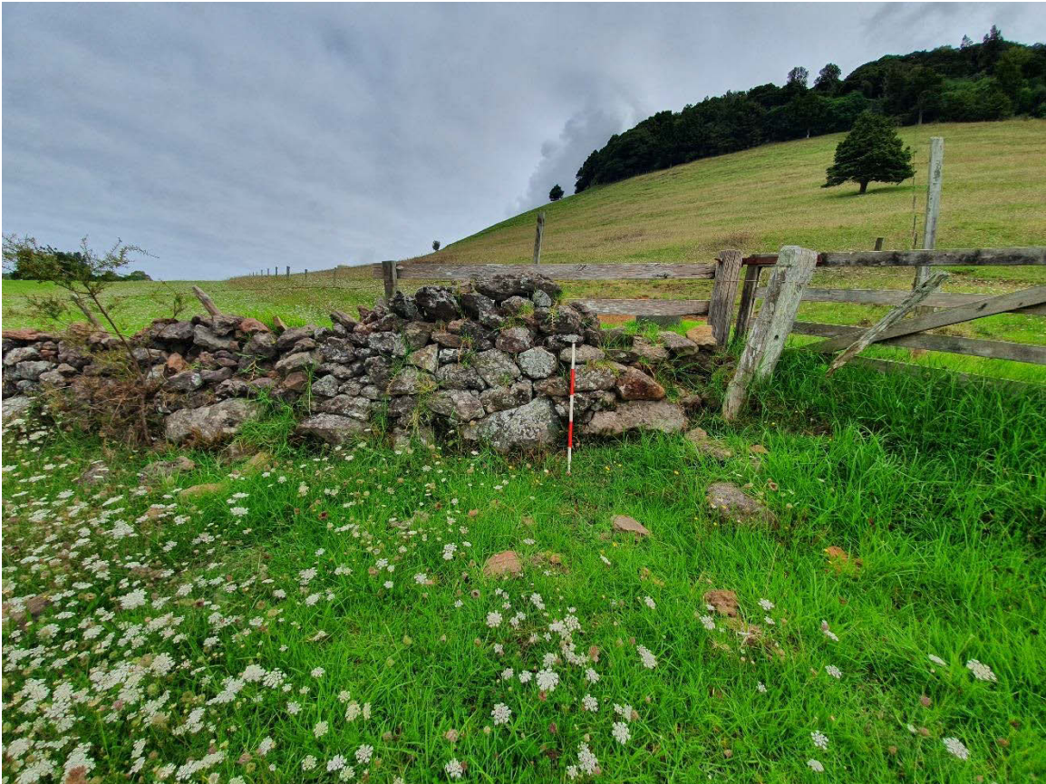
Figure 63: Terminus at north eastern end of stone wall.
