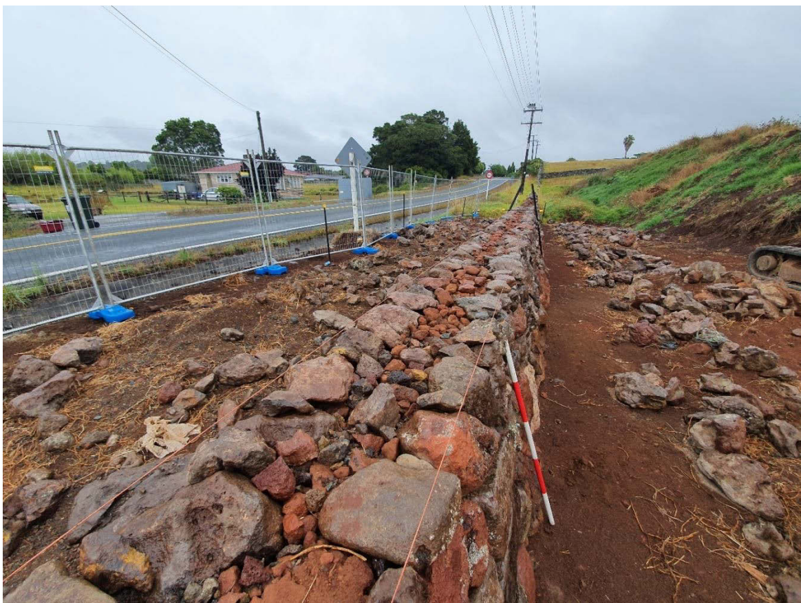
Figure 36: Reconstruction of stone wall.
