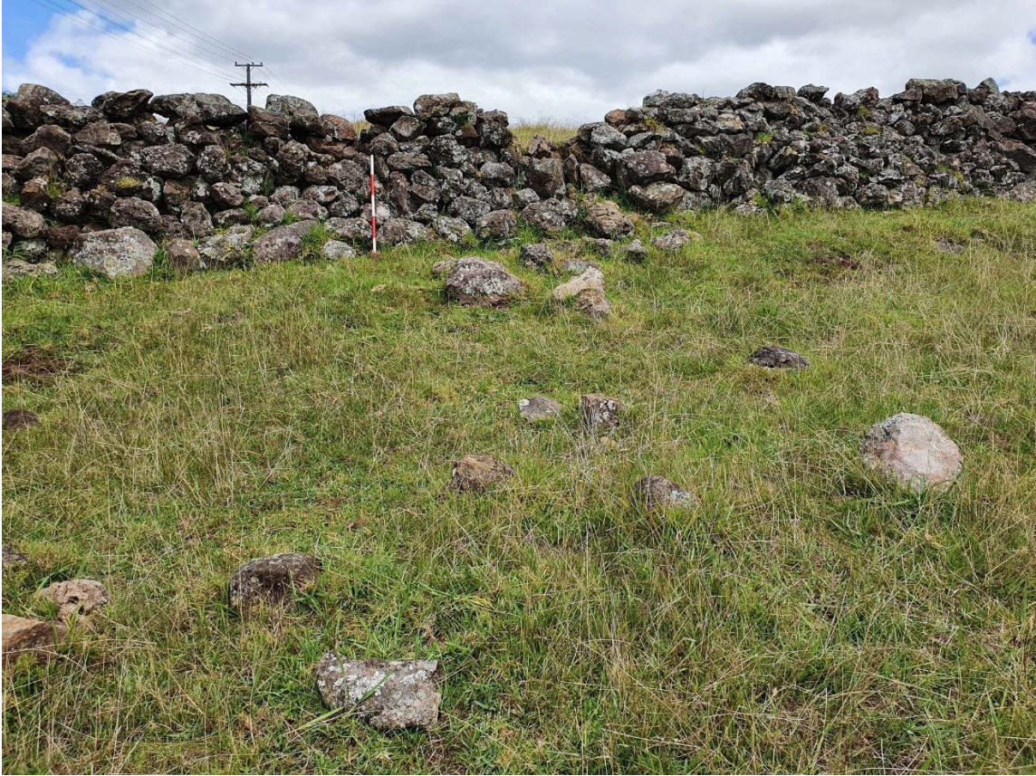
Figure 53: Section of wall in poor condition.
