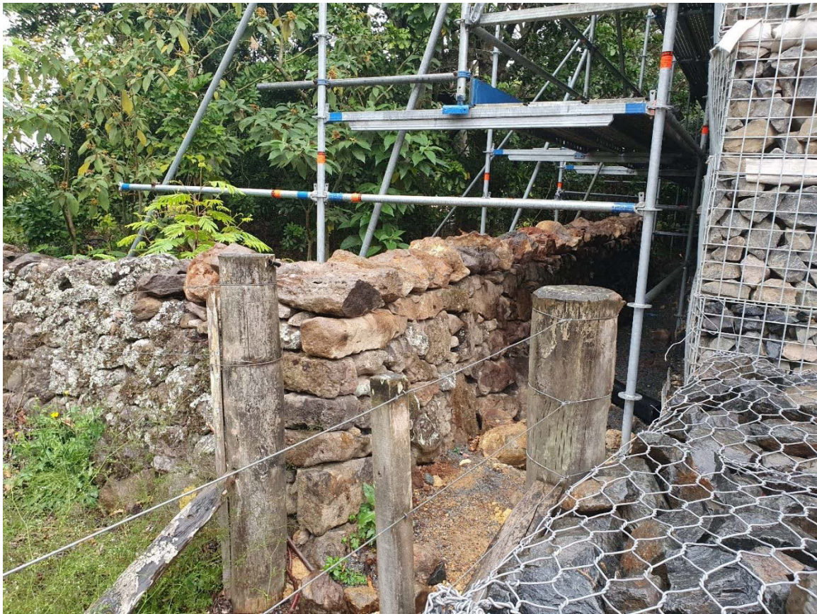
Figure 41: Otapapa boundary wall relocation.
