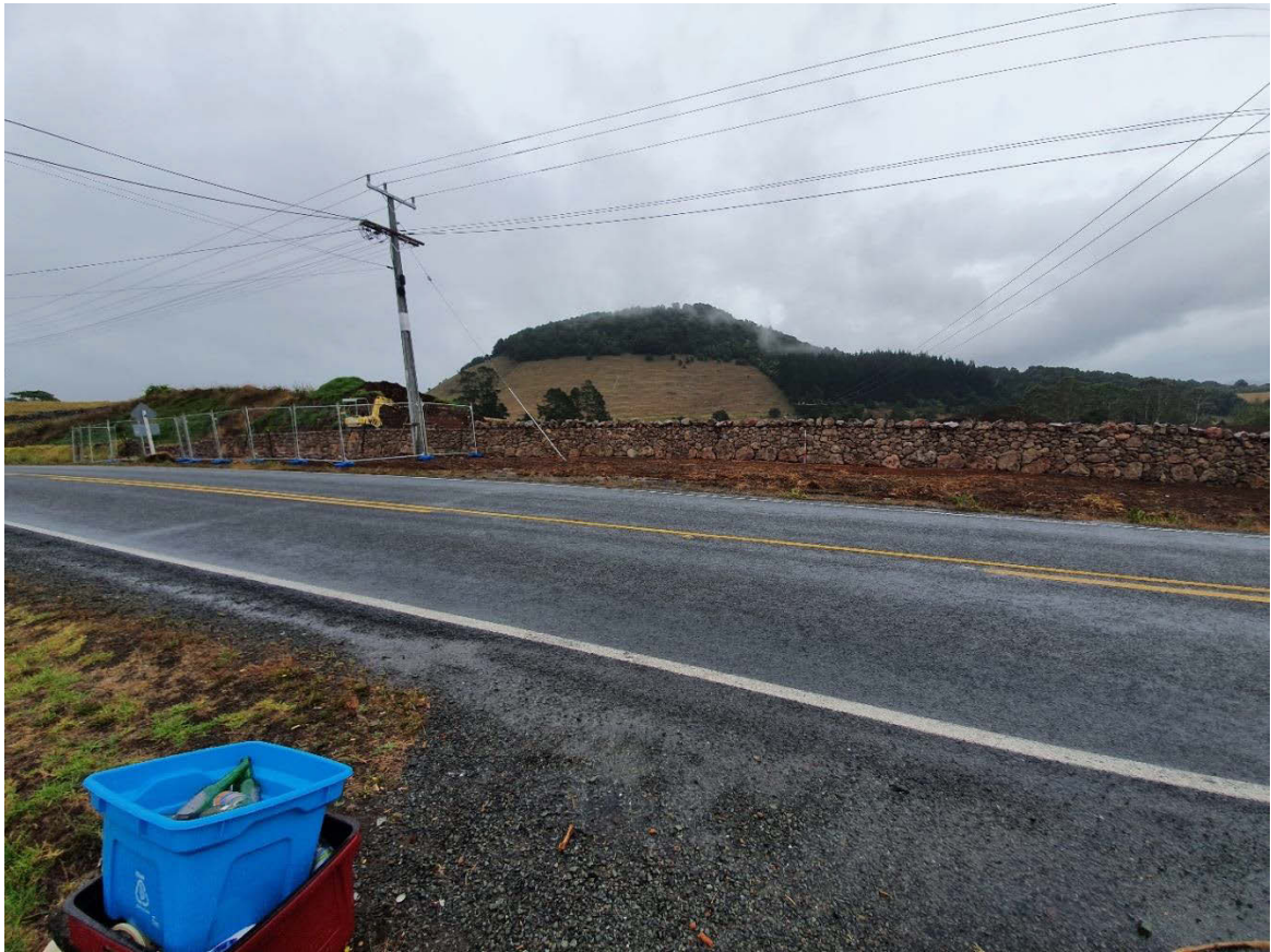
Figure 35: Northern hillock, after re-contouring and relocation of power pole.
