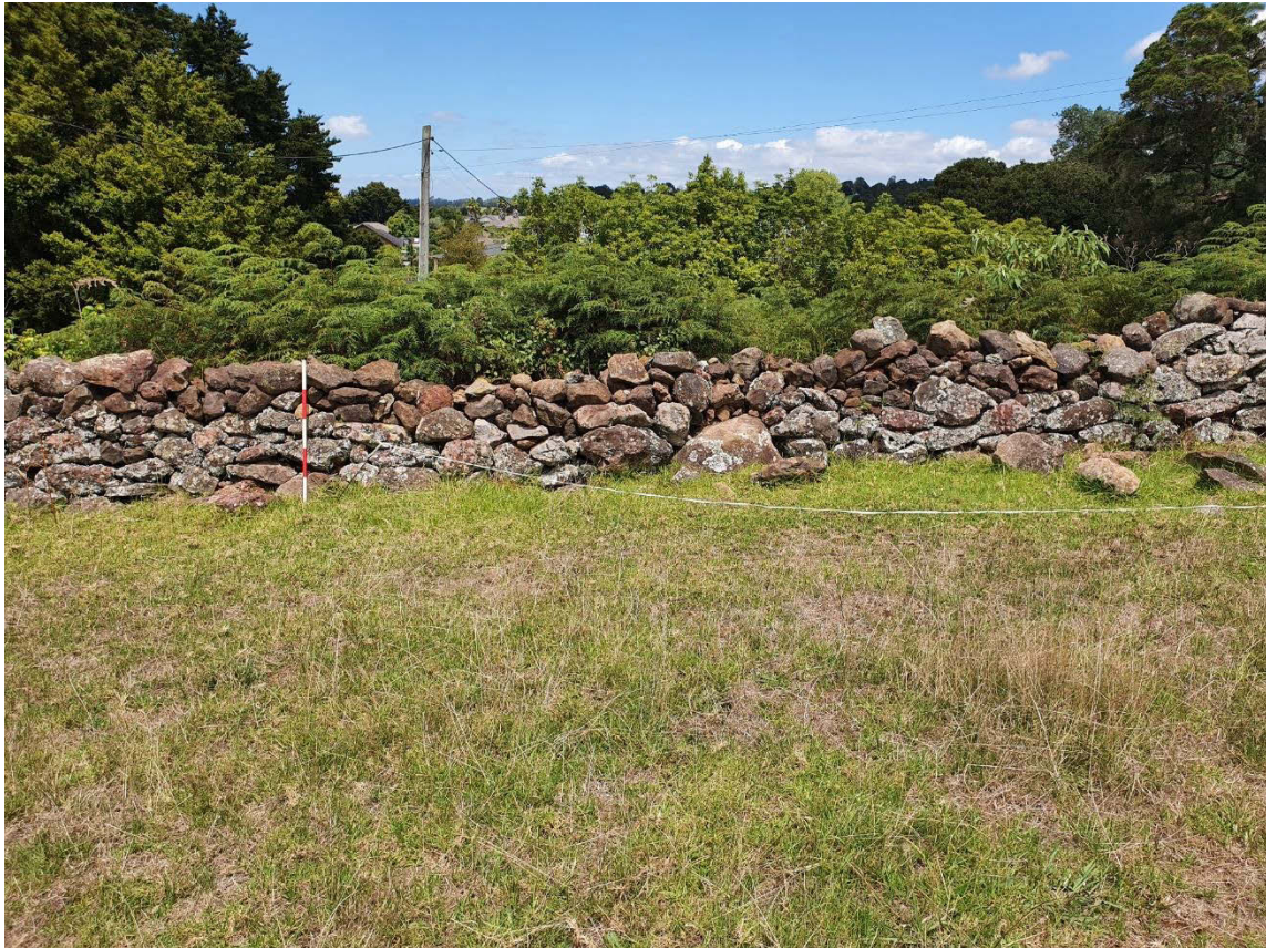
Figure 51; Poorly repaired section of Three Mile Bush Road boundary wall.
