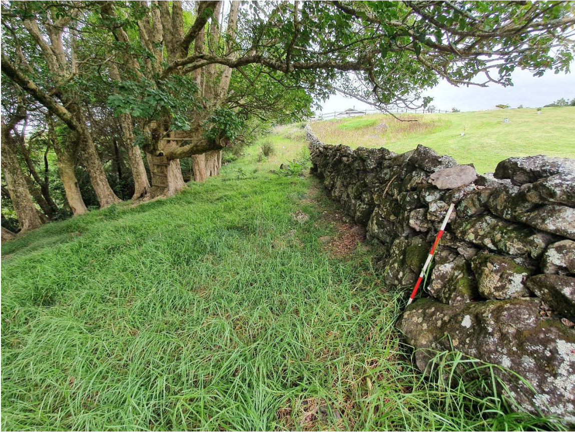
Figure 62: Looking south west along internal wall.
