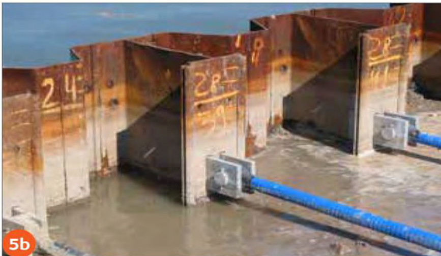
Figure 42: Concept single combi-pile wall with tie back anchors (WSP Concept Design Report, 2022)
