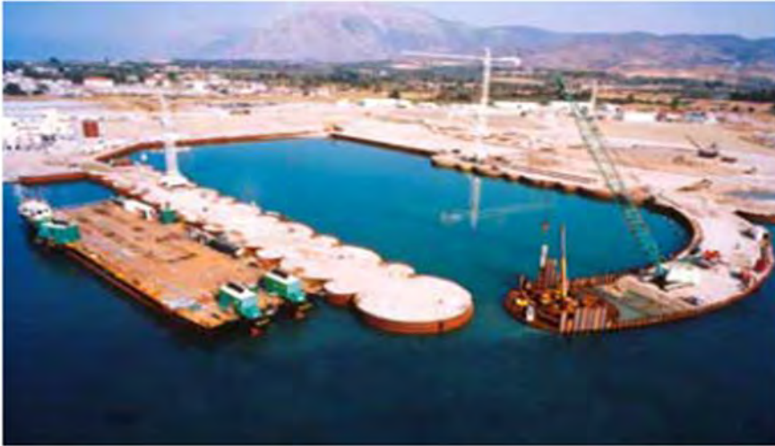
Figure 41: Concept interlocking circular caissons with gravel or sand infill (WSP Concept Design Report, 2022)
