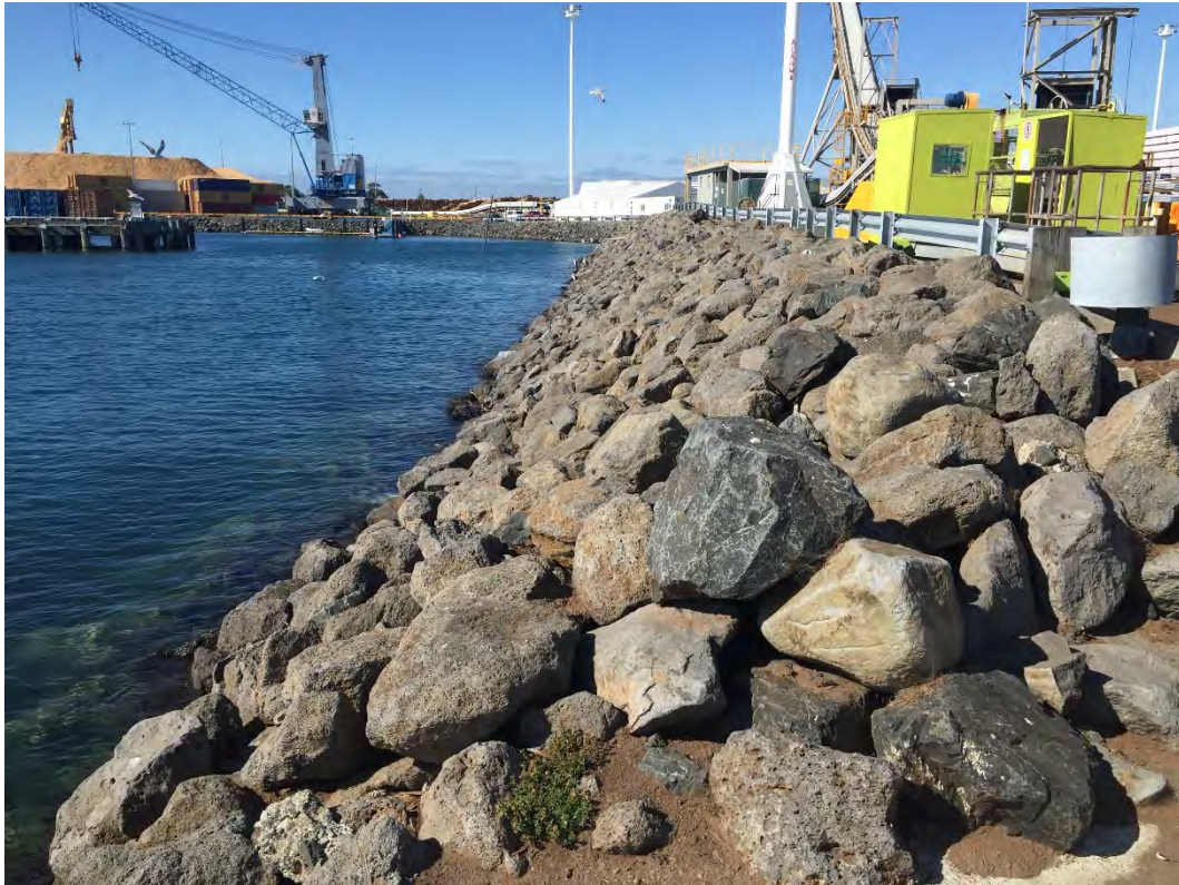
Photo 7: Riprap along the edge of Berth 3
