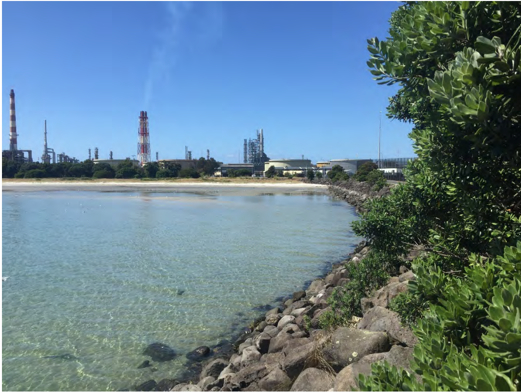
Photo 6: View of the riprap revetment along the eastern boundary of Northport boundary
