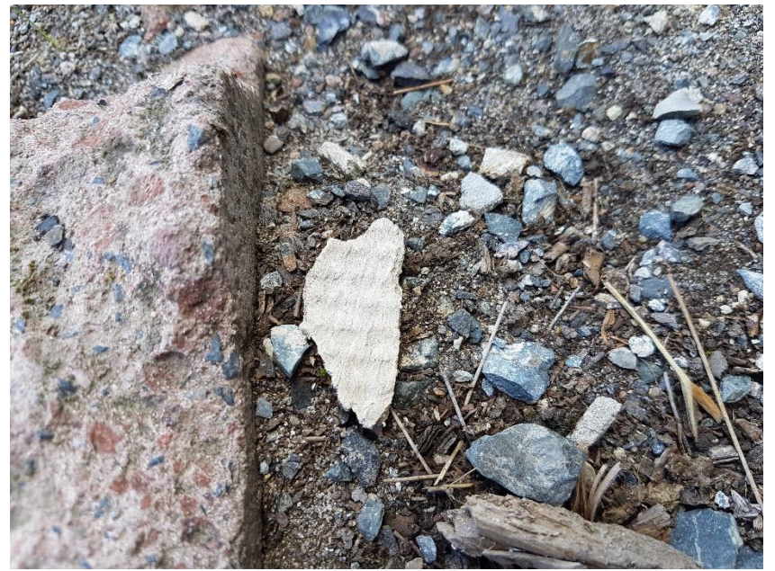
PACM in Soil Around Raised Water Tank
