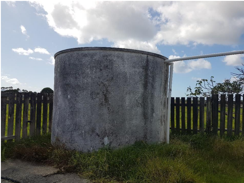
Concrete Water Tank
