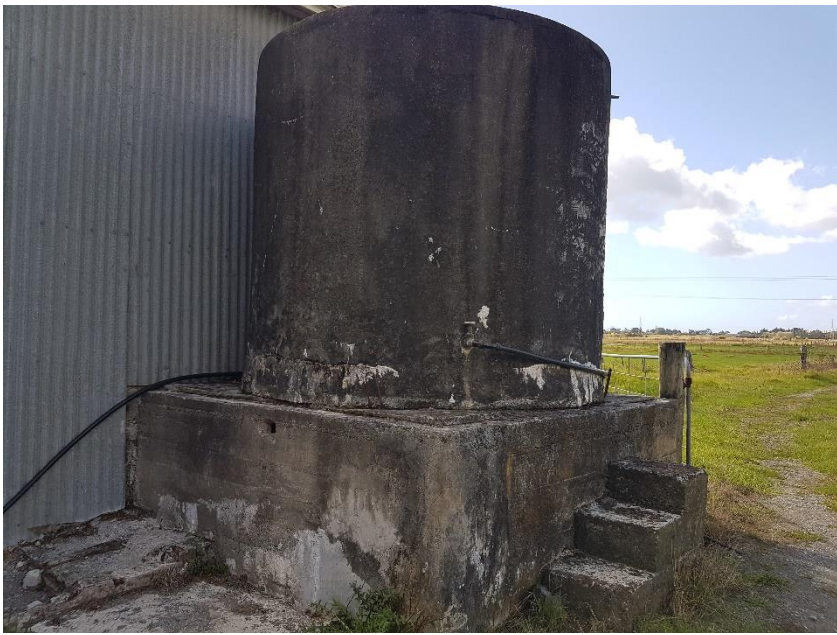
Raised Concrete Water Tank
