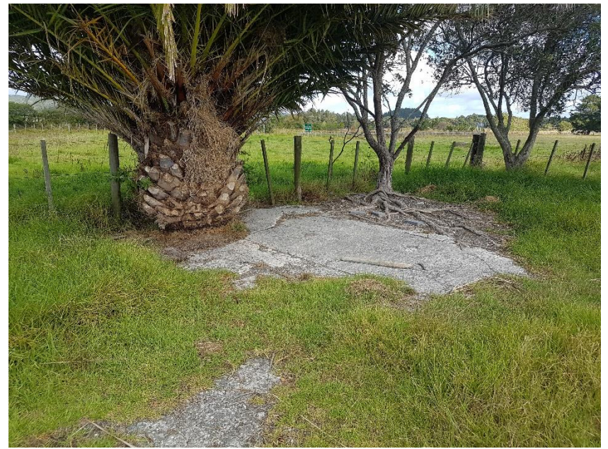
Concrete Building Platform
