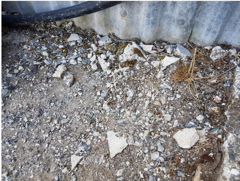
PACM in Soil Around Raised Water Tank
