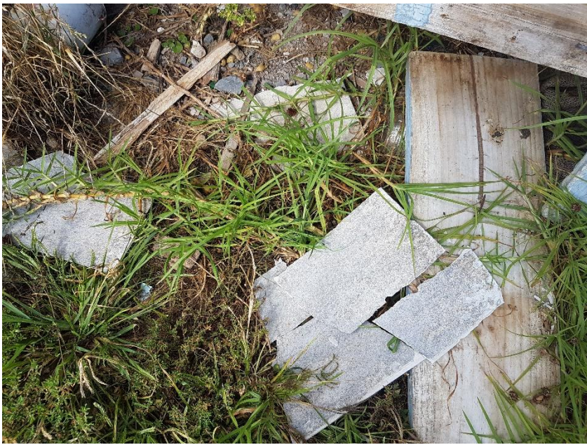
PACM in Soil Adjacent to Dwelling
