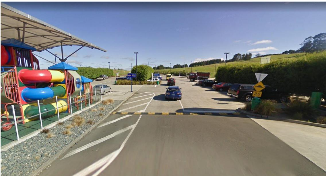
Figure 6: Typical retrofitted speed hump on internal road layout in service centre (Google, 2009)
