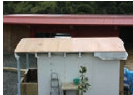
2. Creation of roof deck (plywood over laminated timber beams)
