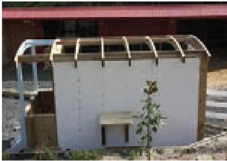
1. Timber roof support structure created (using laminated beams)
