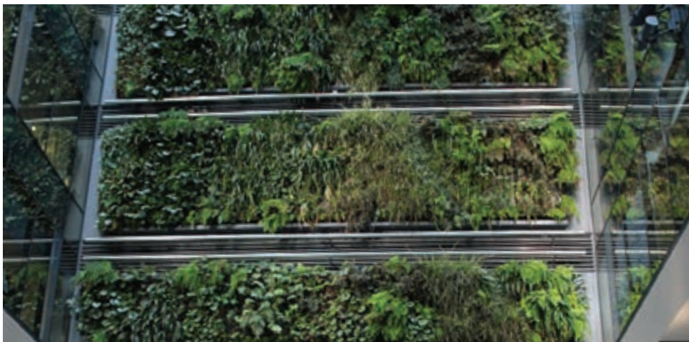
Below: Hydroponic living wall system at The Atrium, Auckland. Photo Sam Hendrikse
