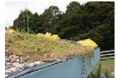
8. Completed living roof installation
