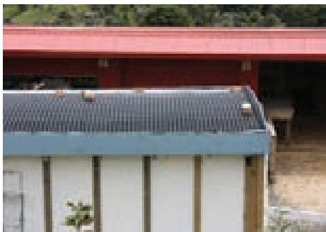
5. Plastic drainage layer placed over pond liner
