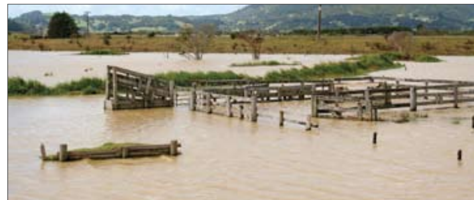
Figure 22: Flood Damage Near Hikurangi, July 2007
