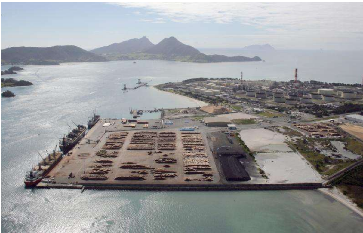
Figure 1. Aerial Photograph of Marsden Point Port
