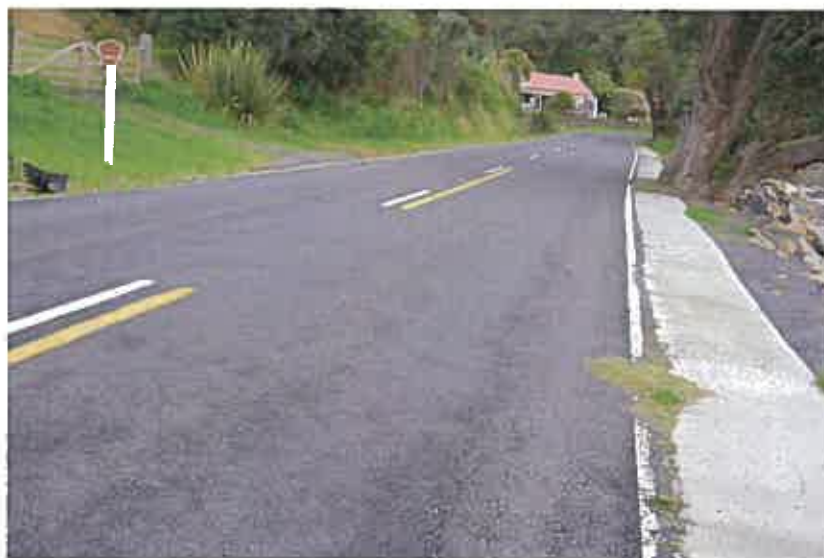
Frontage of Mania Gardens and previously consented land for subdivision, showing foot paths, power, water and sewage services (evidence of ongoing housing in the area to the East).
